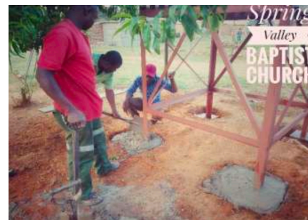
Samuel, Nelson, and Antony installing the water stand.
